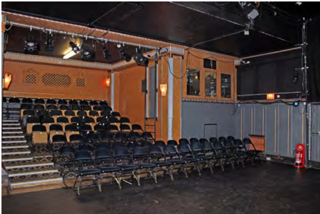
A general shot of the studio, showing the modern overcladding of the walls and soffits and the position of the south and lighting booth
