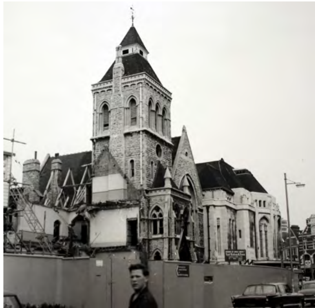
Photograph showing the Town Hall during the demolition in 1968
