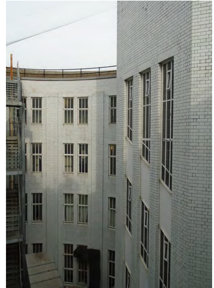
A view of the stairwell showing the distinctive glazing bars
