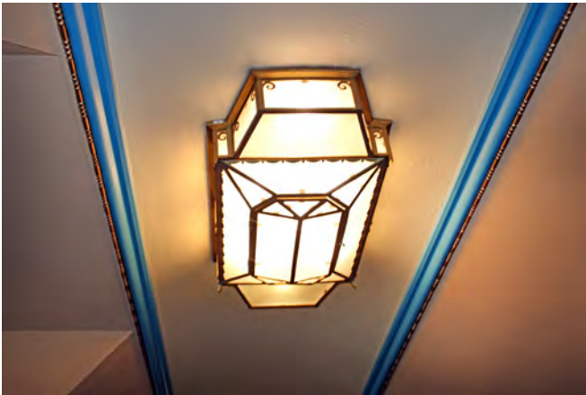
FF2: Art deco metal light fitting fixed to ceiling
