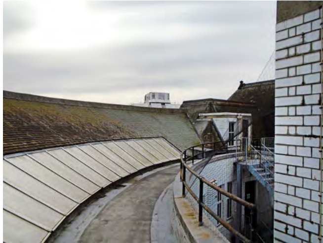
Views across roof facing south-west
