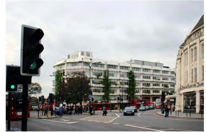
The A21 as it curves round the building, defines its setting to the south and east
