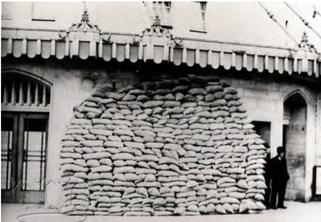
Photograph showing sand bags outside the Broadway Theatre during the years of the Second World War. Source: Lewisham Archives
