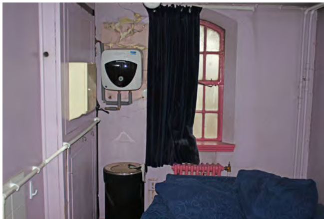
FF4: One of the Dressing Rooms on the first floor
