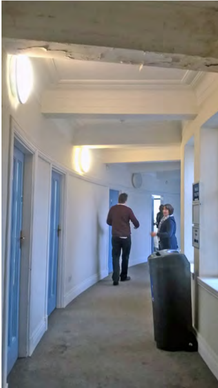
A corridor on the third floor
