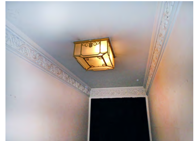
Highly decorative cornices in the secondary circulation space within the Broadway Theatre building
