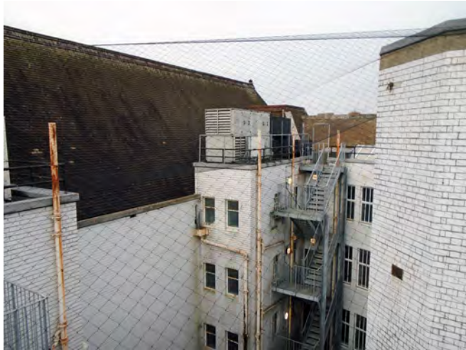
Views across roof facing north-west
