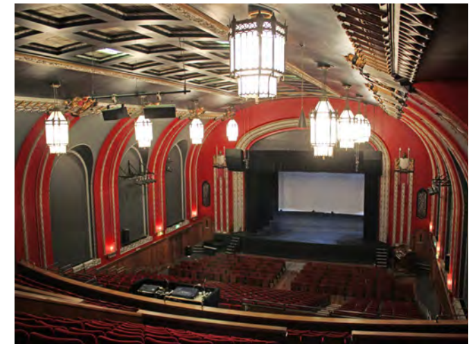
Ceiling fixed light fittings within the concert hall
