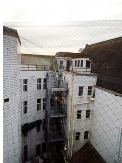
Views across roof facing south
