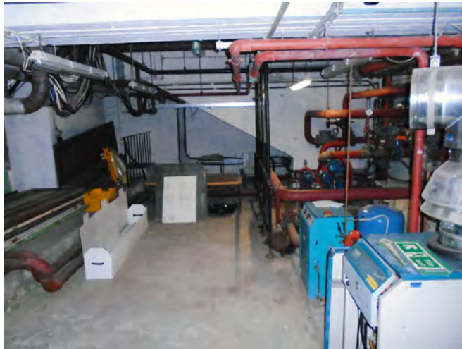
Basement plant room
