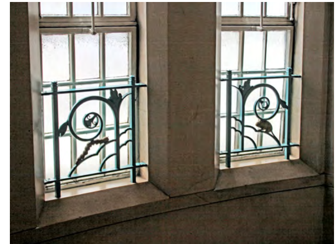
Internal decorative metal work to the lower portion of the window openings
