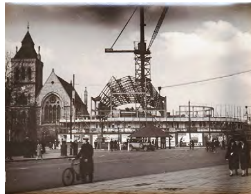
Construction of Lewisham Town Hall Extension 1930
