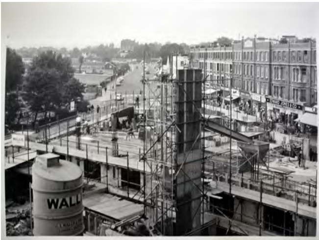
The Civic-Suite mid construction, 26th September 1961. Source: Lewisham Archives
