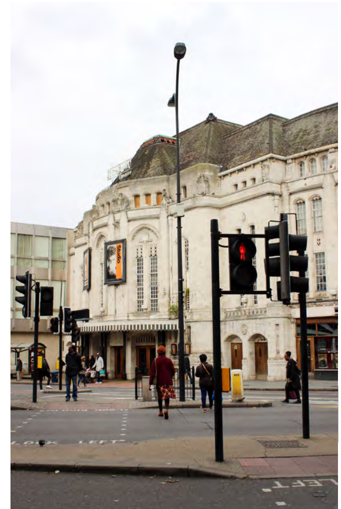
Pedestrian crossing in front of the Broadway Theatre southern elevation
