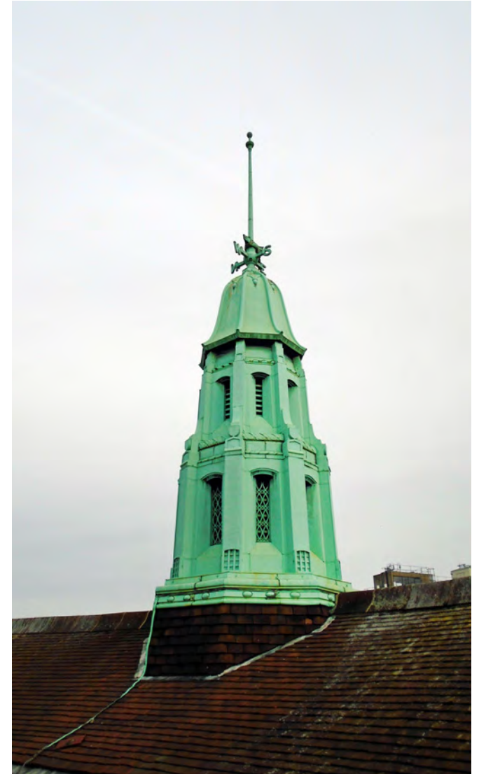
Two-storeyed steeple to the east side of the roof
