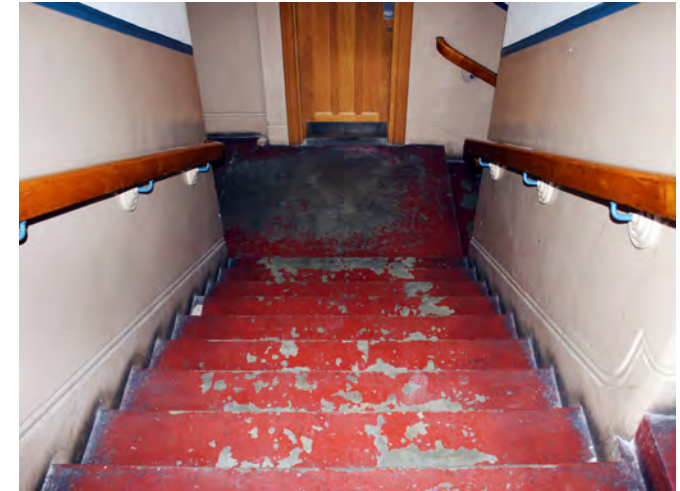
Deteriorated floor finish demonstrated in the back of house circulation space
