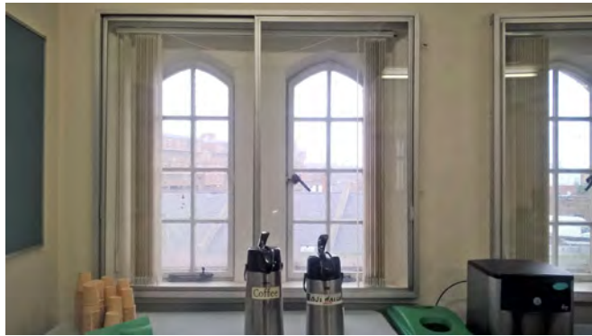
Cloze-up on the secondary glazing on the second floor
