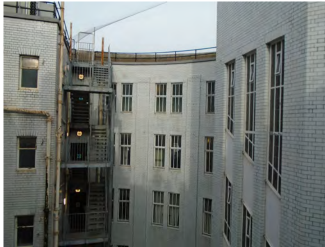
A view of the glazed bricks in the lightwell looking north
